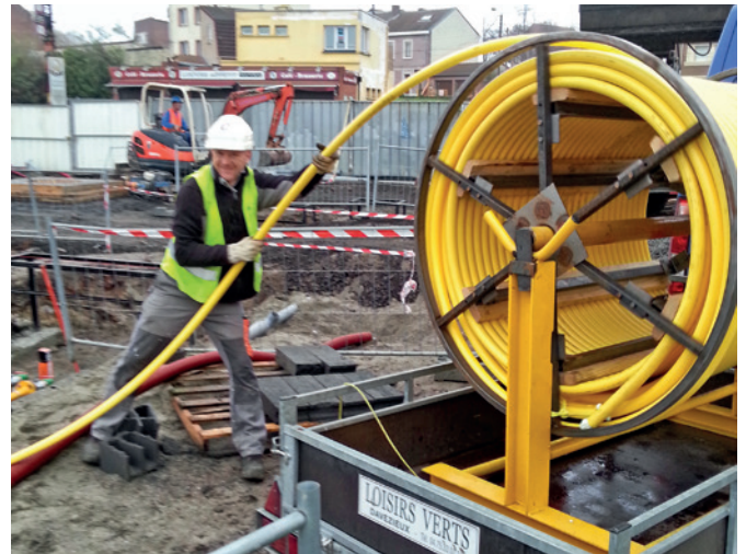
Installation of pipe LPG-FLEX
